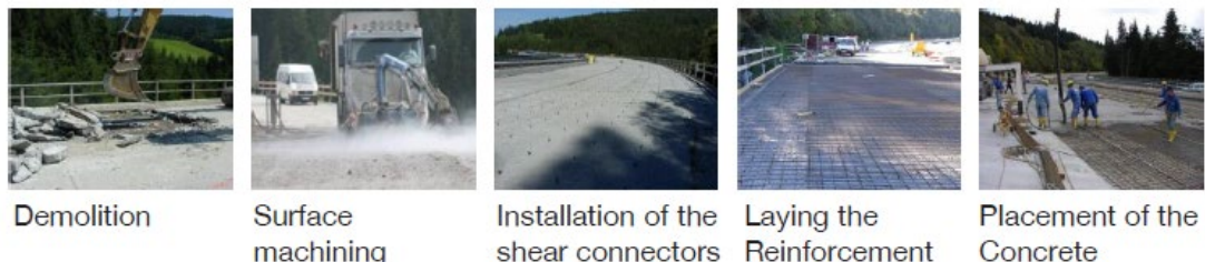
Fig. 10: Construction of concrete overlays
